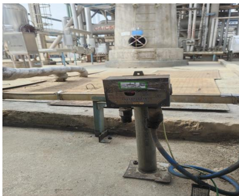
池体泄漏检测设施
