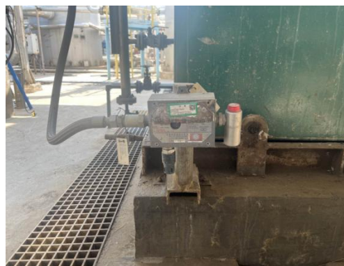
池体泄漏检测设施
