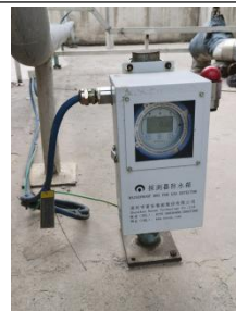
池体泄漏检测设施
